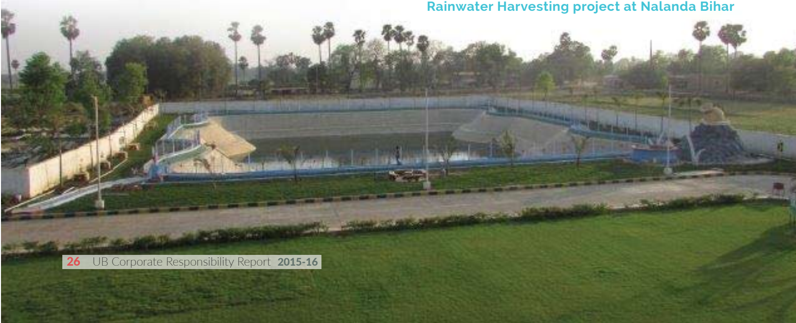
Rainwater Harvesting project at Nalanda Bihar
