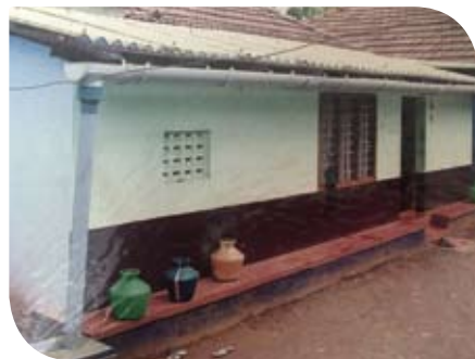
Rainwater Harvesting at Ganeshapuram, Palakkad
